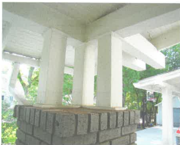
Square, wooden columns on a brick pier
