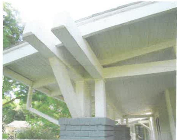
Columns, rafters, and bracing exposed
