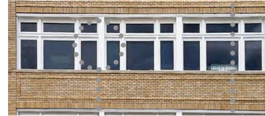
GROUPED WINDOWS 208 E Louisiana St
