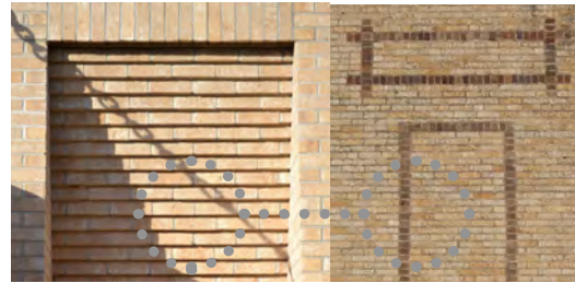
INSET BRICK PANELS 107 1/2 E. Virginia Parkway
