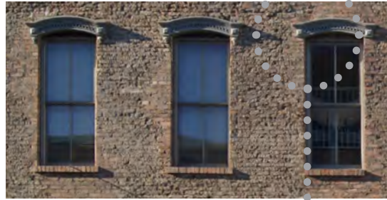
ARCHED WINDOW HEAD DETAILING 228 E Louisiana St
