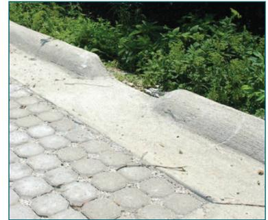
**Figure 4.** Curb cut opening.
