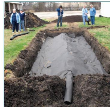
Figure 6. Placing the filter fabric.
