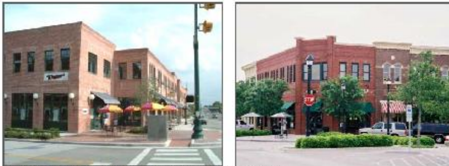
Images illustrating acceptable exterior building materials
