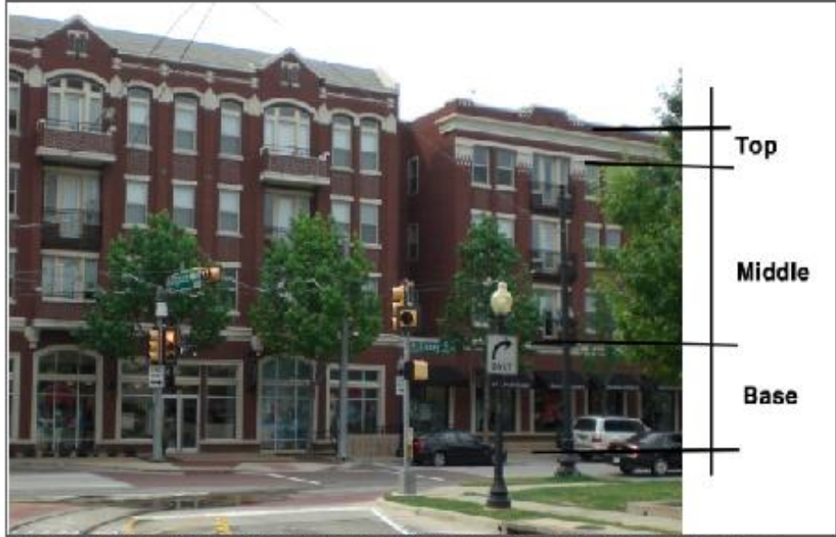
Image illustrating simple and rectilinear building form with a clear base, middle, and top
