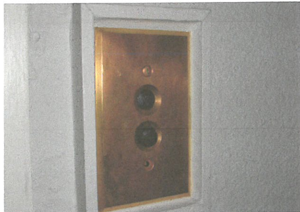
Brass switch plate is framed by molding.
