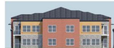
North Elevation - 82% Masonry (51% Brick, 31% Stone, 18% Stucco)
