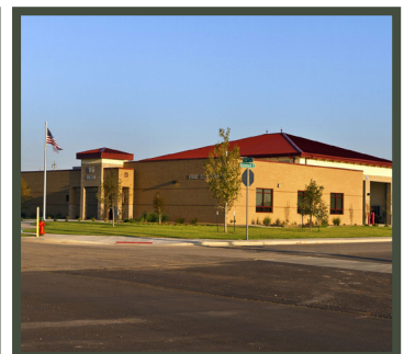
City of Lubbock Fire Station No. 16, Lubbock, Texas
