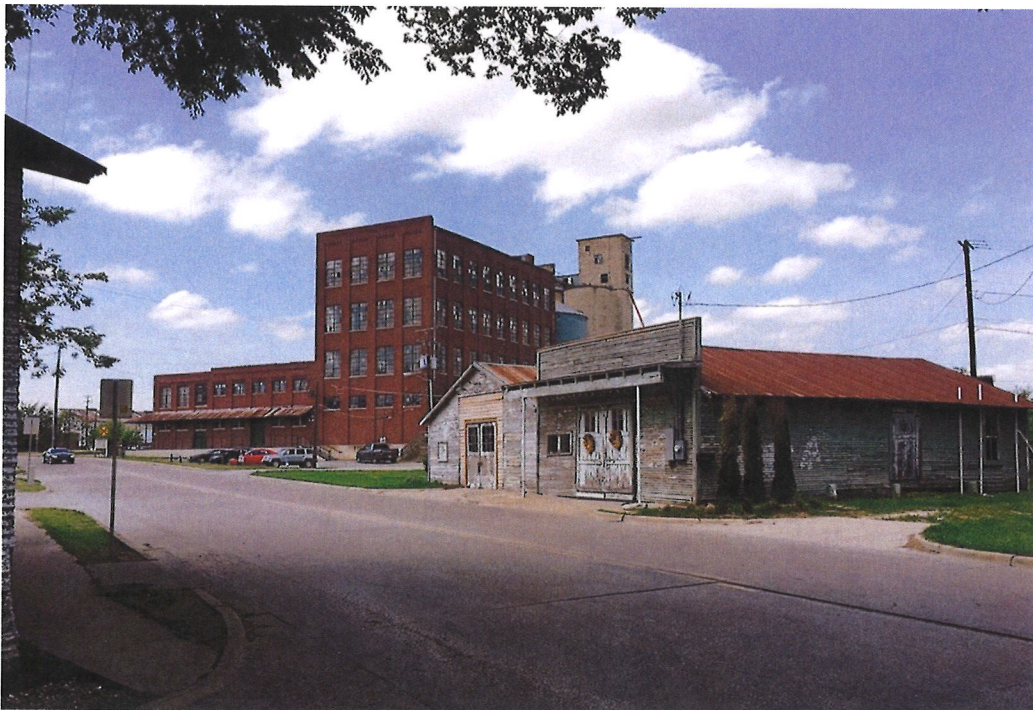
705 Greenville Road, as purchased. (photo taken prior to any work being completed)
