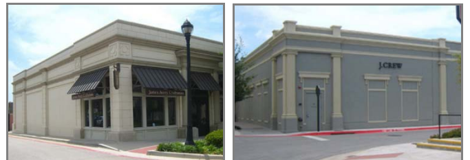
Images showing the side and rear façades buildings finished to match the color and materials of the front facades
