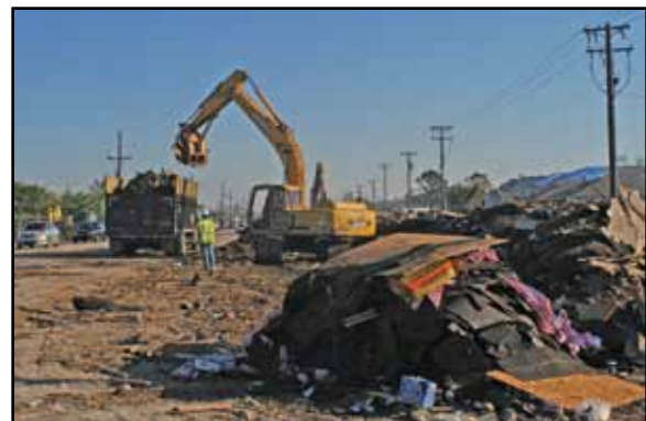
Figure 1: Contractor debris operation
