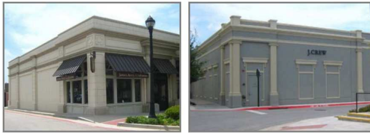
Images showing the side and rear facades buildings finished to match the color and materials of the front facades
