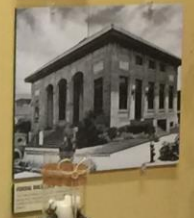
COLLIN COUNTY PRISON The Collin County Prison was built in 1850 and was the first prison in McKinney. The prison was destroyed by fire in 1880 and was replaced by the current building in 1881.
