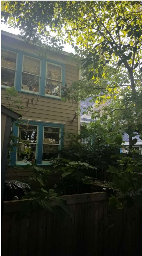
Back Elevation: North East facing
