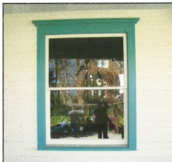
One-Over-One sash windows
