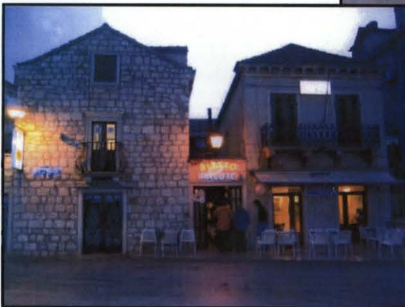
Windows have a vertical proportion in shape and detailing. Stone masonry will be used with stucco and other quality materials.
