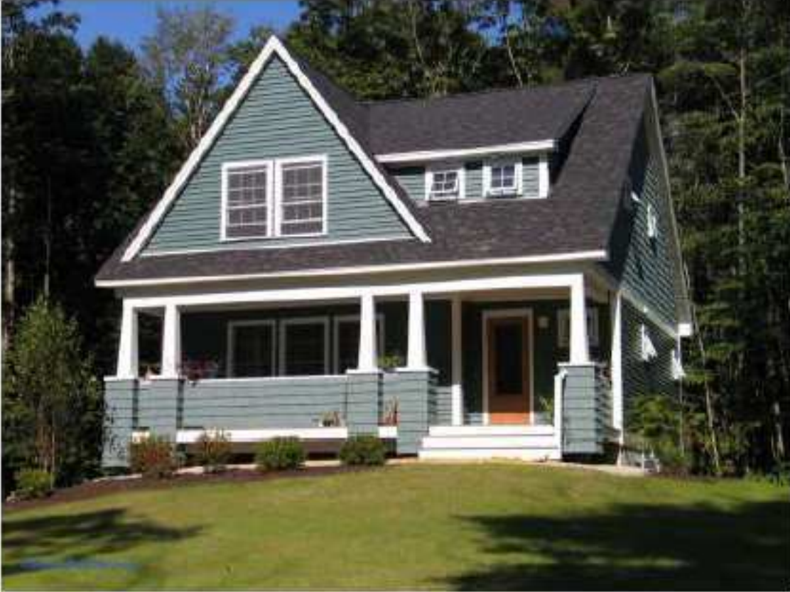
Colonial Revival Twist Style Architectural Example
