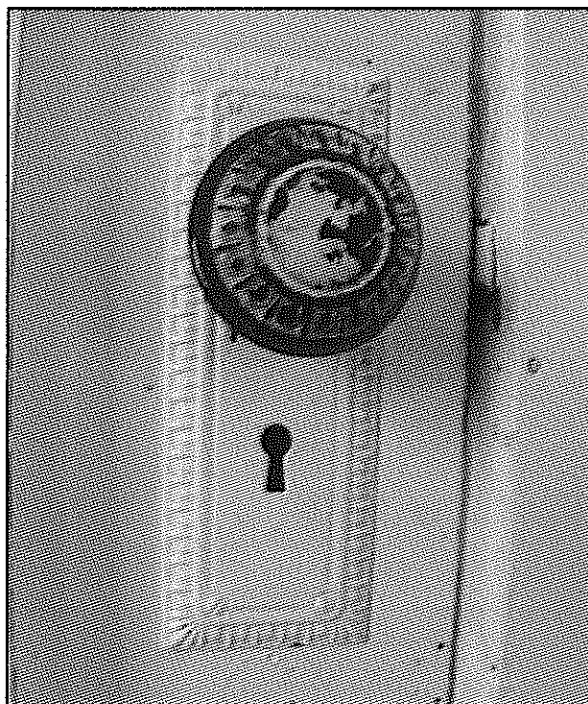
The original door knob remains on the front door.
