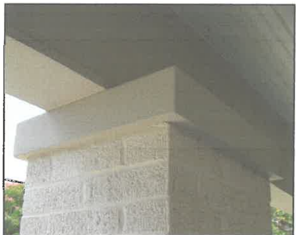
Plain limestone cap on brick column
