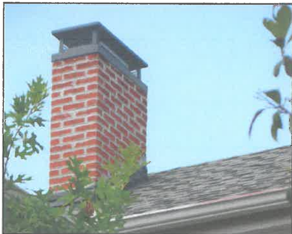
Chimney made of "carpet" brick
