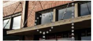
AWNINGS CUSTOMIZED TO REUSE BRICK 304 W Virginia St
