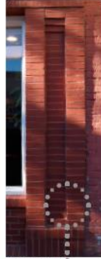
BRICK PLASTER DETAILING 303 E Virginia St
