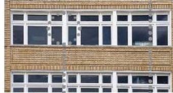
GROUPED WINDOWS 308 E Louisiana St
