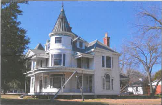
1206 West Louisiana Street
