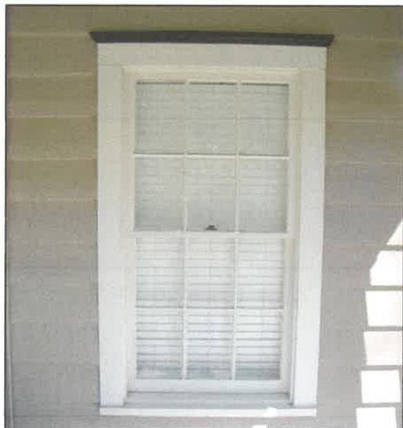
Six-over-six sash windows
