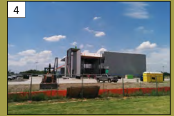
Life Fellowship Church 6400 Henneman Way Valuation: $4.7 million Permit Issuance: February 2016
