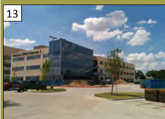
Baylor Scott & White Medical Office (Bldg 2) 2550 W. University Dr. Valuation: $8.9 million Permit Issuance: November 2015
