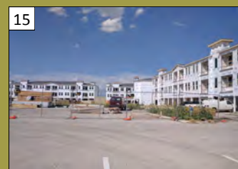
Raleigh House 4450 S. Ridge Rd. Valuation: $31.5 million Permit Issuance: October 2015
