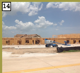
14 Townplace Suites by Marriott 1832 Marketplace Drive Valuation: $3 million Permit Issuance: April 2013
