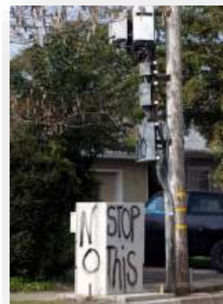
Recent Example of Poorly Managed Wireless Infrastructure Deployments
