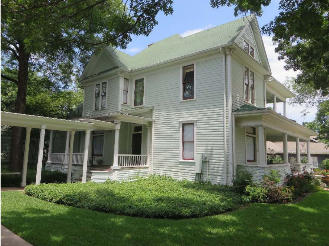
Current photographs of house: west side and back
