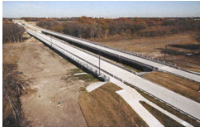
Figure 123 Example of a basic bridge: Hardin Bridge McKinney, TX
