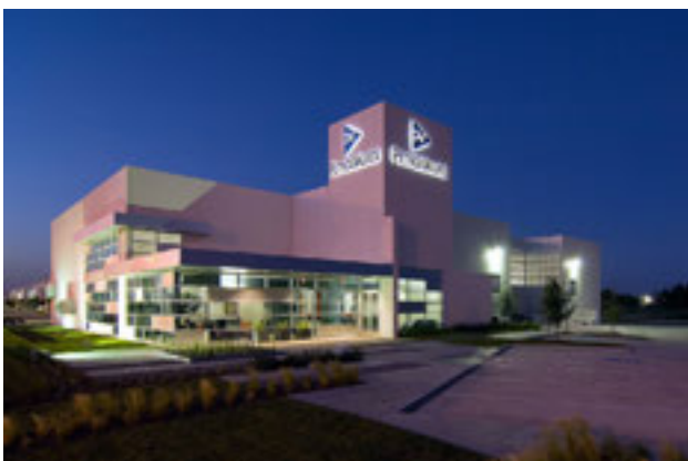
Figure 56 PetrolValves , Powers Brown Architecture
