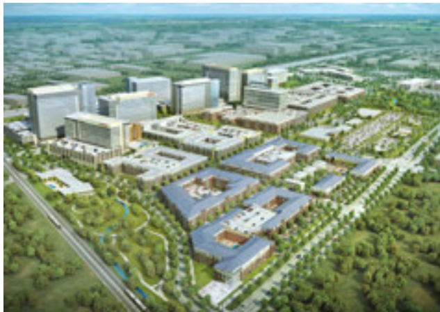
Figure 74 An example of building heights along a regional highway that transitions to less intense development Image Credit: KDC. CityLine DFW. Richardson, TX
