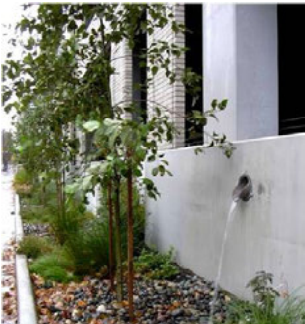
Figure 45 Example of drainage alternatives: downspout
