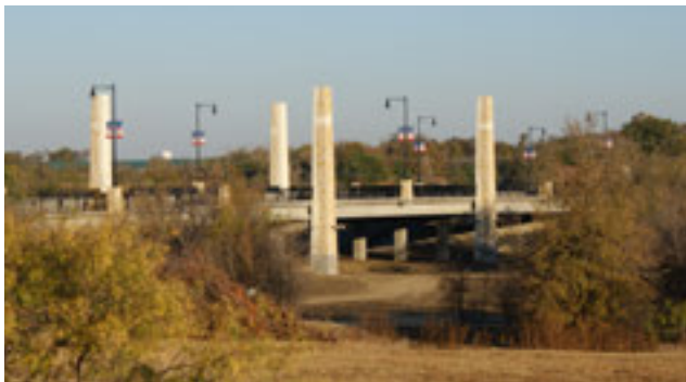
Figure 124 Example of a gateway bridge: Witt Road Bridge Little Elm, TX
