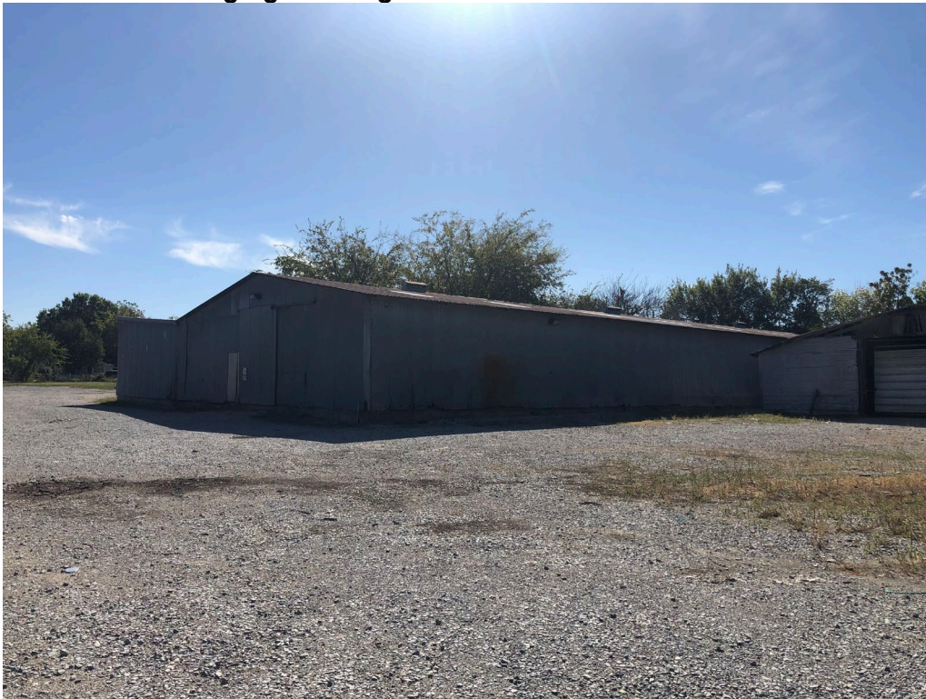
Photo of Barrel Aging Building
