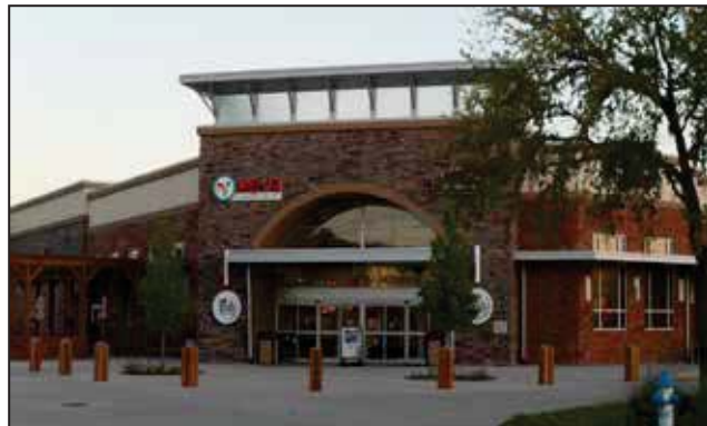
Figure 4.09.03.4: Building with Sheltered Entry
