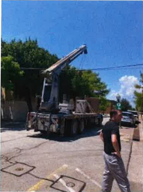
FLATBED USED TO DELIVER GREASE TRAP FIRST TIME. DRIVEN BY PRECON PRECAST LLC EMPLOYEE. SNAPPED POWER LINE AND TELEPHONE POLE IN DOWNTOWN MCKINNEY.
