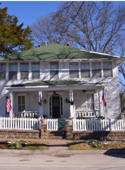
Picket on retaining wall
