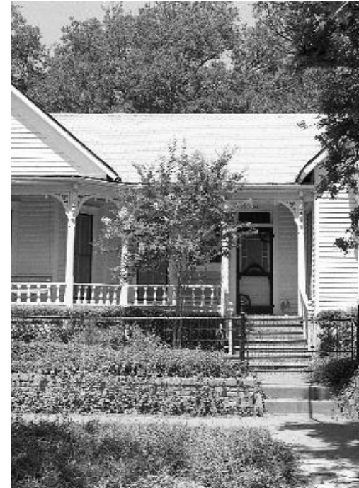
Metal on retaining wall
