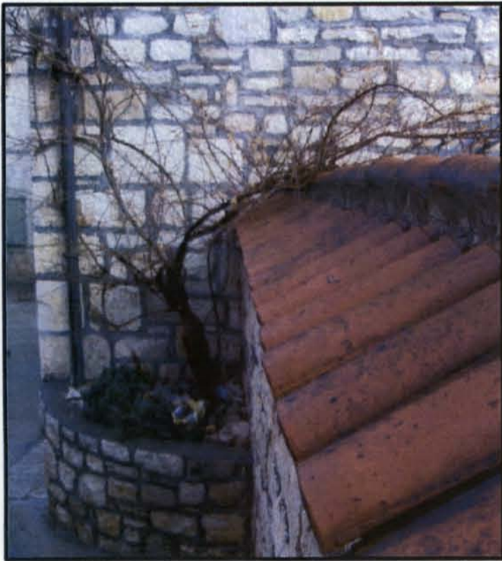
Stone walls, decorative wrought iron railings, and red clay tile roofs will be used in the village architecture. Strategically placed plantings will soften the appearance of buildings.
