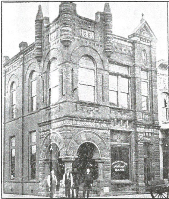
Collin County National Bank, Est. 1881
