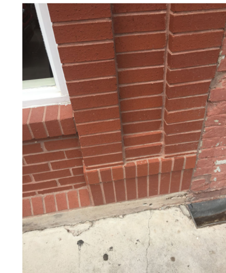
3 brick column detail scale: nts
