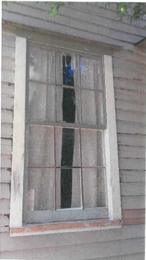
Exterior Window during work
