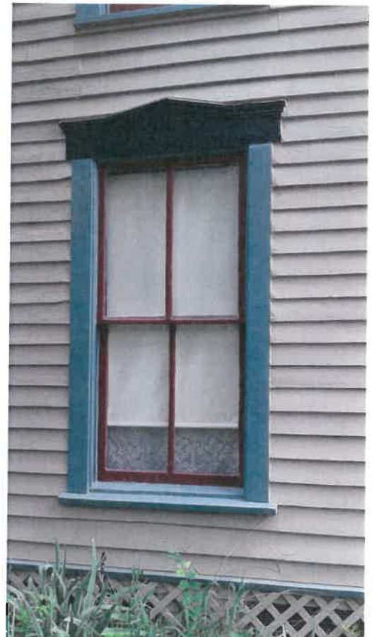
Repaired and repainted window
