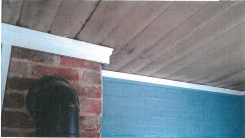
New exposed shiplap ceiling in kitchen
