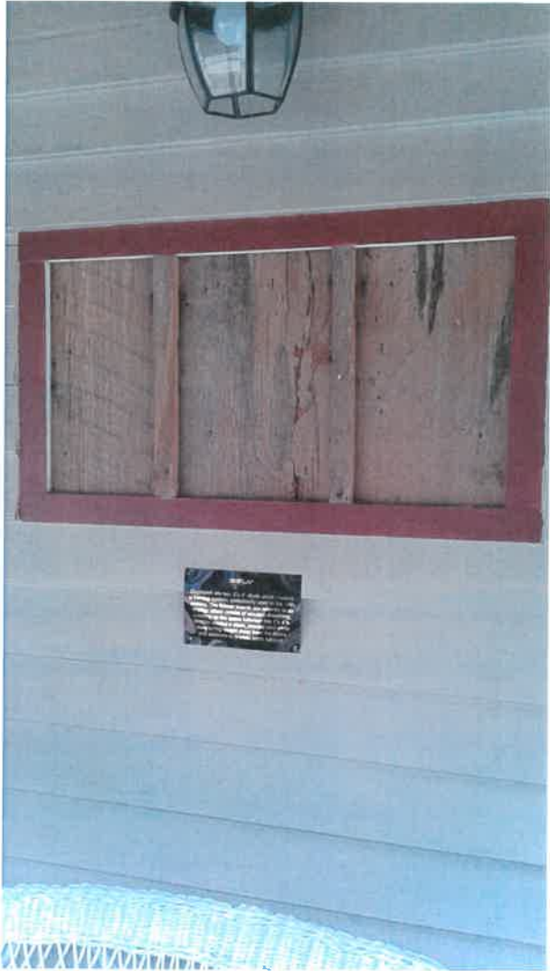
Exposed shiplap with explanation of structural use
