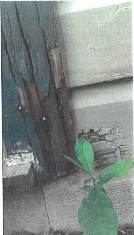
Damage to Visitors Center caused by above ground sprinkler heads in flower beds
