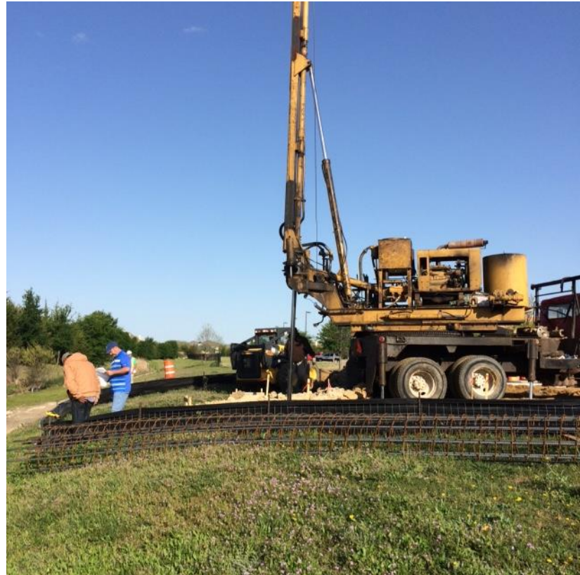
Drilling for bridge piers
