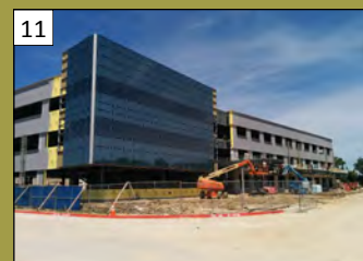
11 Baylor Scott & White Medical Office (Bldg 2) 2550 W. University Dr. Valuation: $8.9 million Permit Issuance: November 2015
