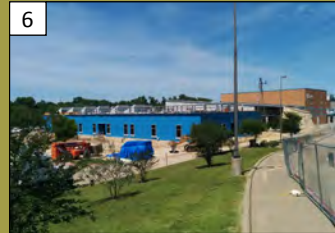
6 Malvern Elementary (MISD) 1100 Eldorado Pkwy. Valuation: $2.6 million Permit Issuance: January 2016
