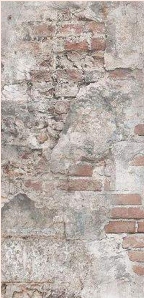
PLASTER LAYERING ON BRICK
