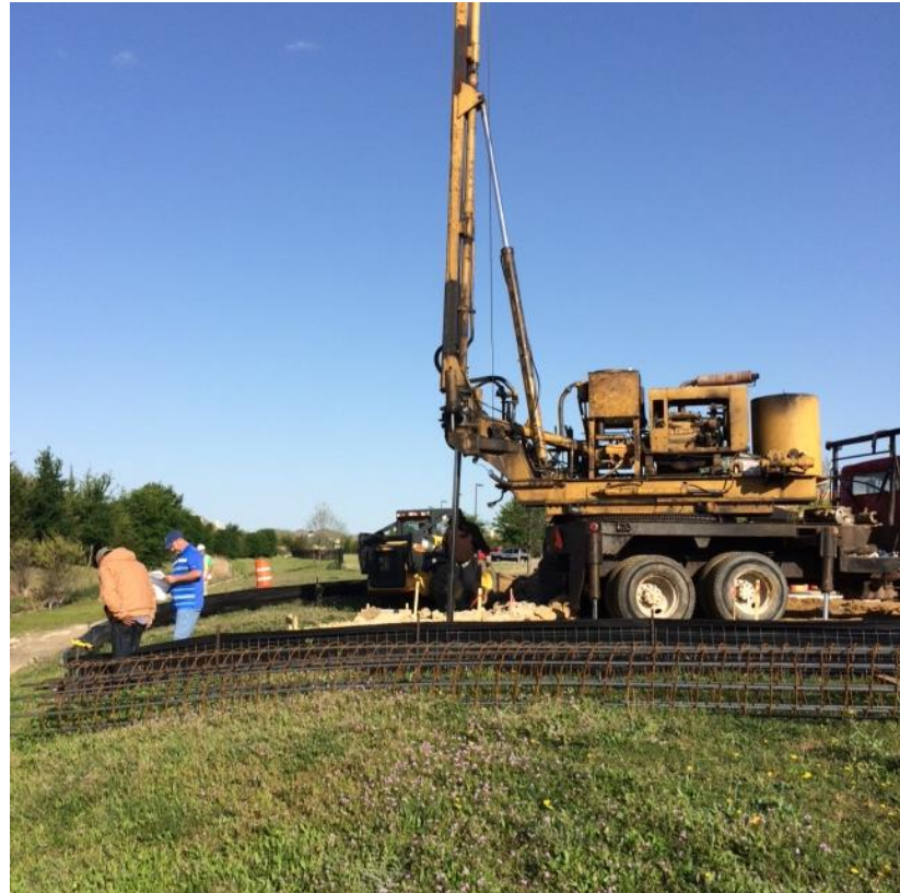
Drilling for bridge piers
