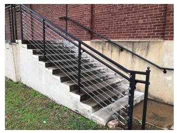
Additional work would include replacing an exterior wood stair with new concrete stairs and railings.
