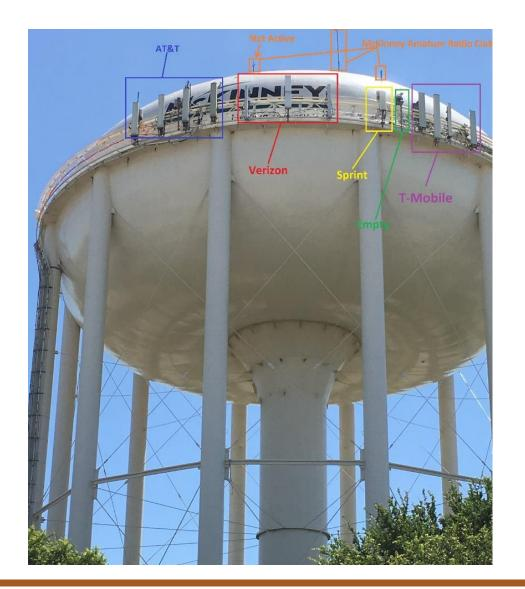
Elevated Storage Tanks are used as towers for communication providers
