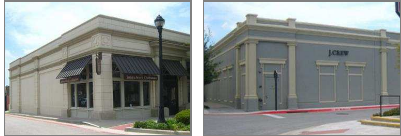
Images showing the side and rear façades buildings finished to match the color and materials of the front façades
