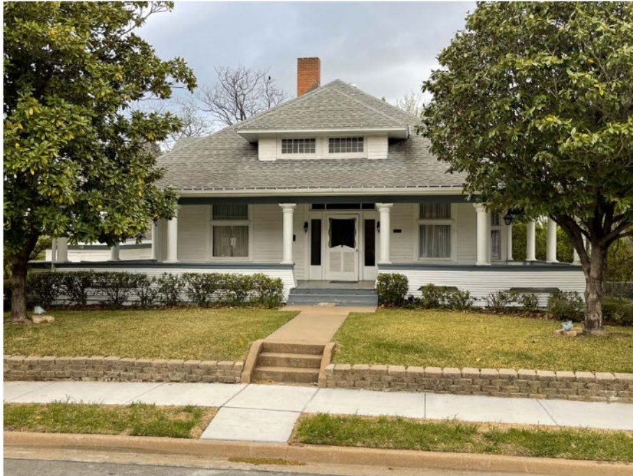
Above: façade Right: north elevation
