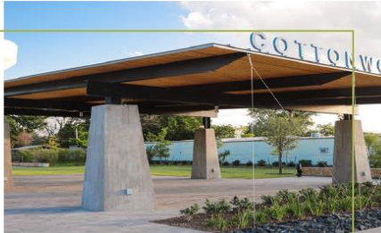
Cottonwood Park Pavilion After
