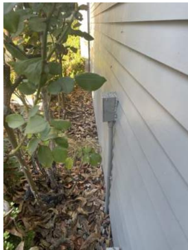
705 N College St #5 (Garage Drainage).
