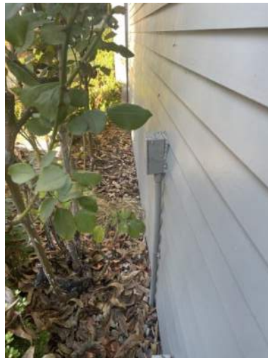
705 N College St #5 (Garage Drainage).
