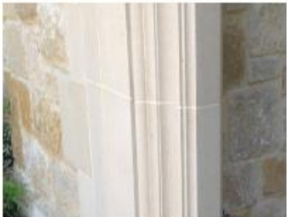
FRISCO BUFF LUEDERS (MASONRY AT DOORS & WINDOWS)
