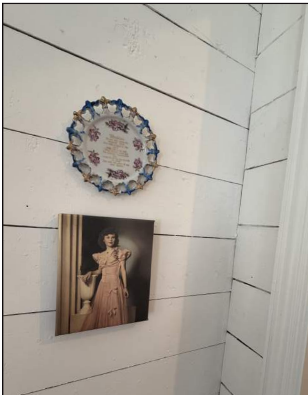
Plank Wall Paneling Exposed
