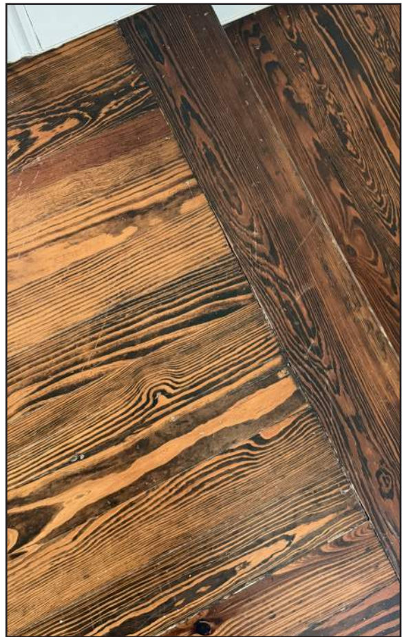
Southern Yellow Pine Flooring on Stairs
