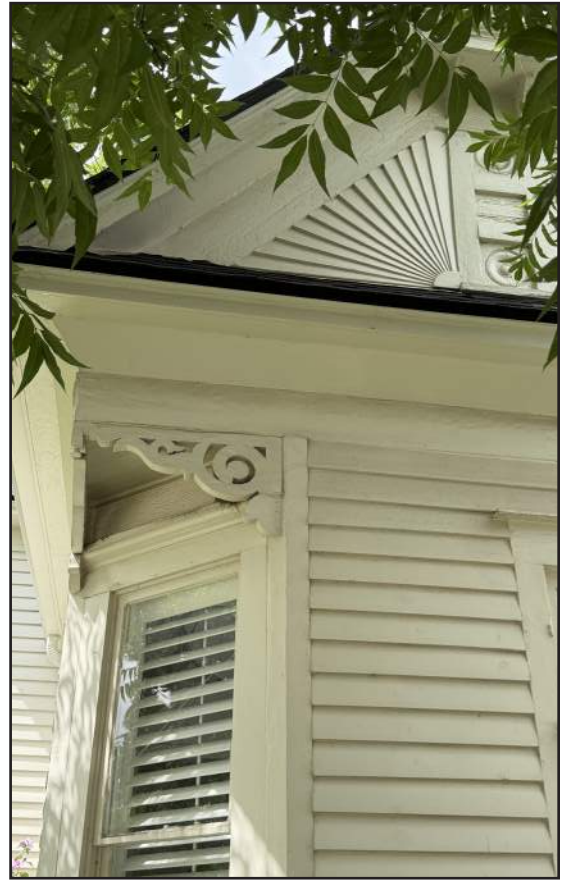
Exterior Queen Anne Detailing
