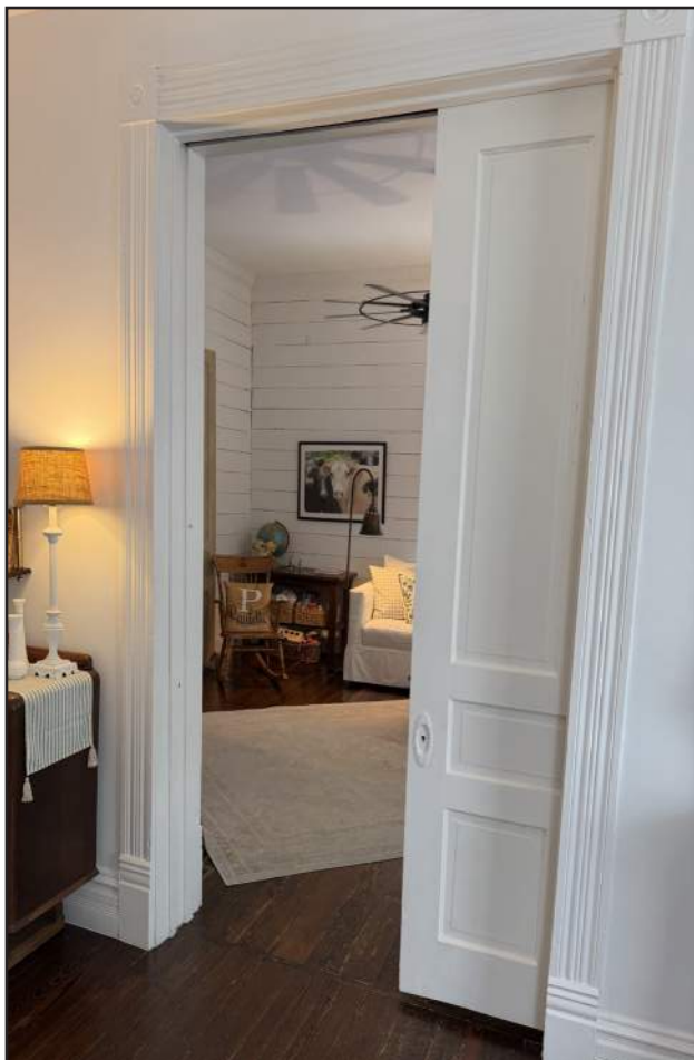
Sliding Pocket Door between Foyer and Living Room
