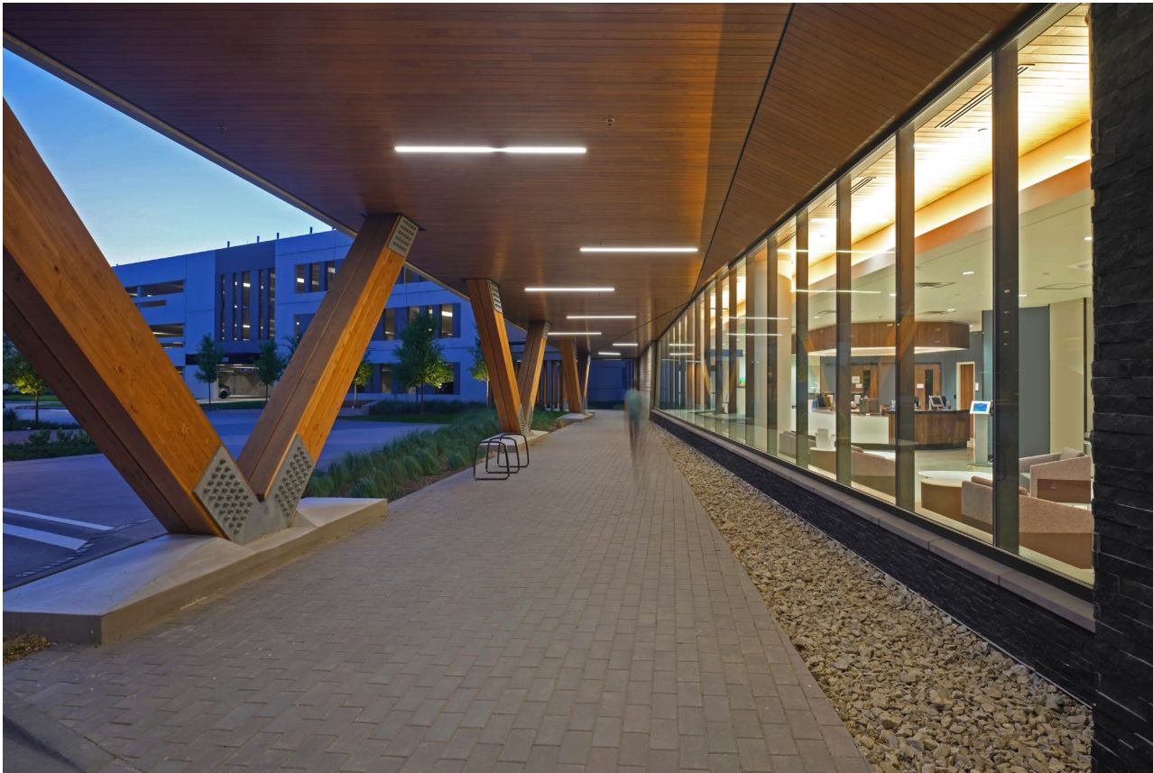
Texas Health Frisco Hospital – Glue Laminated Mass Timber Columns
