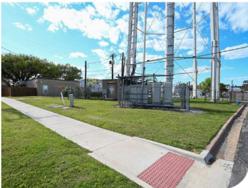
Existing View of Chestnut Tank
