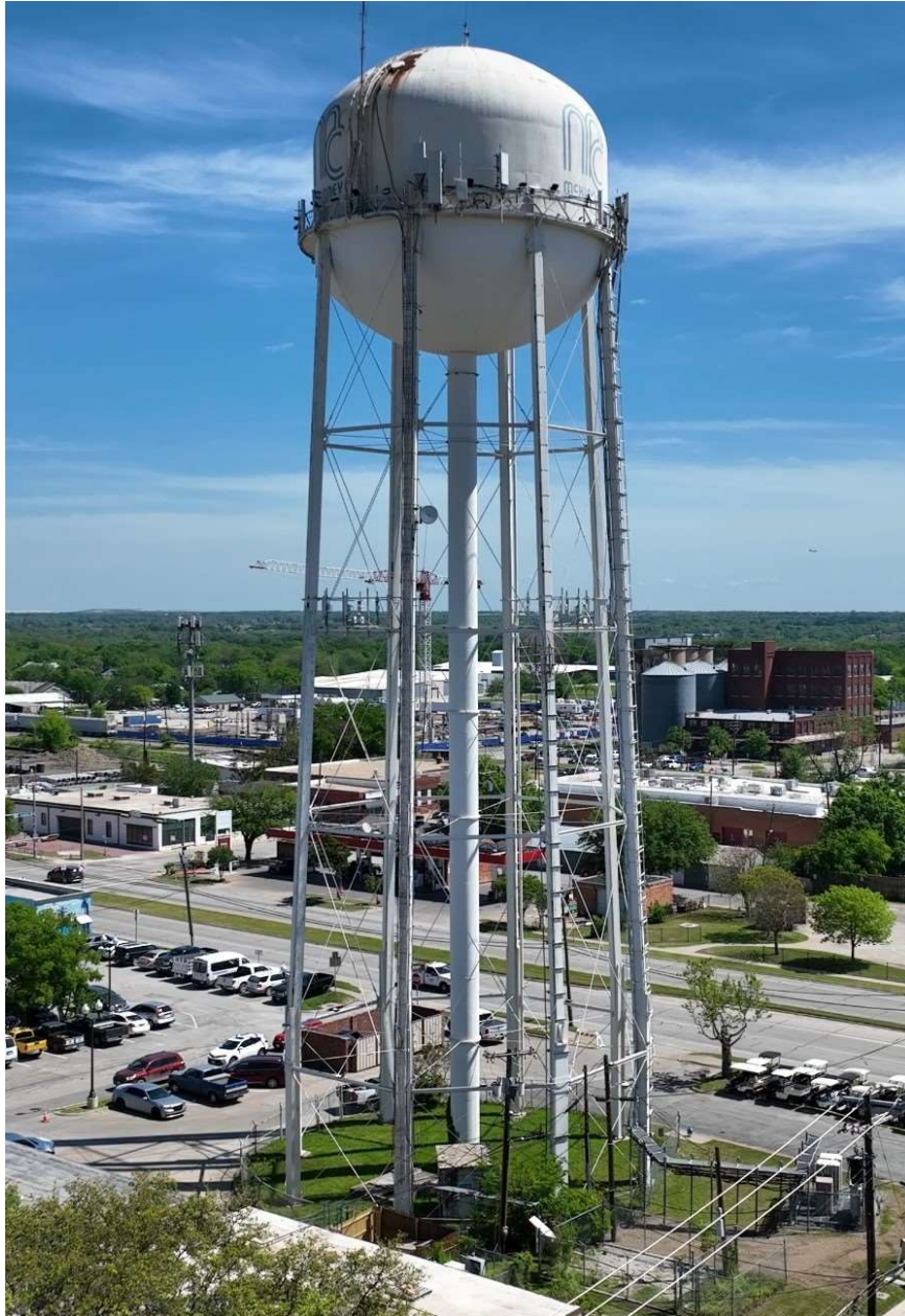
Existing View of Chestnut Tank
