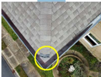
Shingle damage
