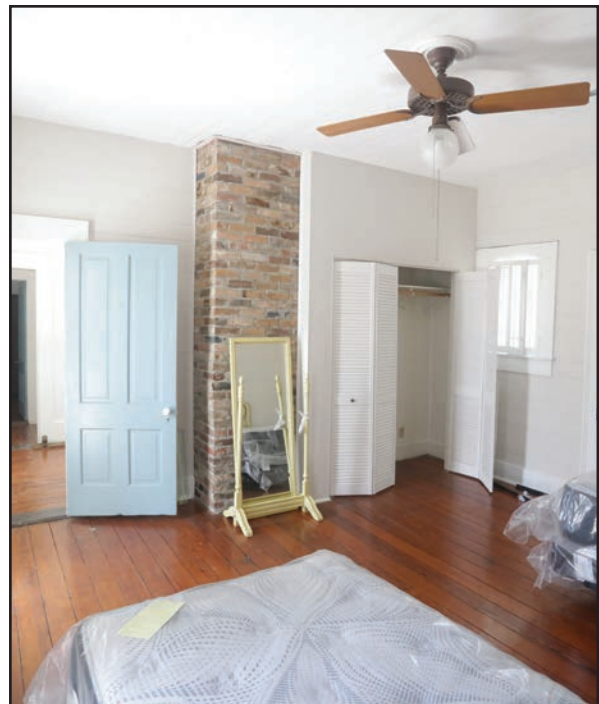
Brick flue from first-floor fireplace
