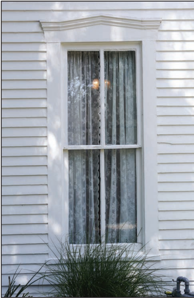
Segmented gable pediment above window
