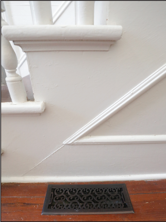
Floor heating vent
