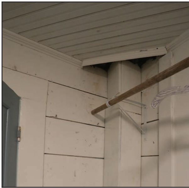
Wallboard planks of original bathroom converted to a closet
